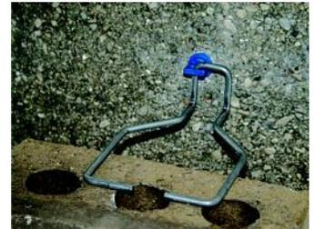
1. Place carbide bit into Condriive 500 drill adapter and tighten set screw. Place drill adapter into chuck of a hammer drill. Drill hole a min. of 1/4" deeper than thread length of SureTie Tapcon.
